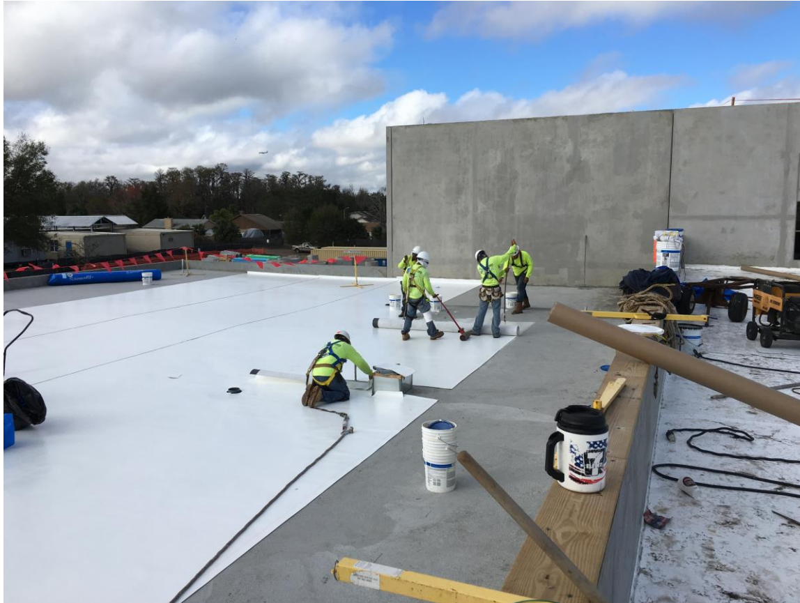
Roofing Membrane Installation
