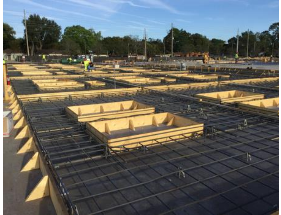
Tilt Panel Rebar
