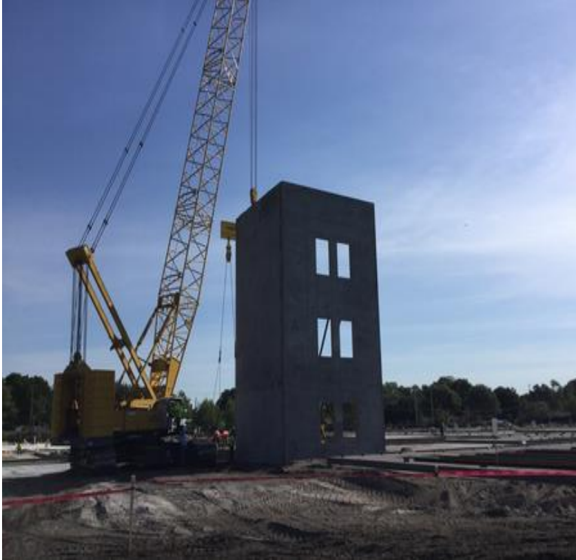
Tilt Panel Erection
