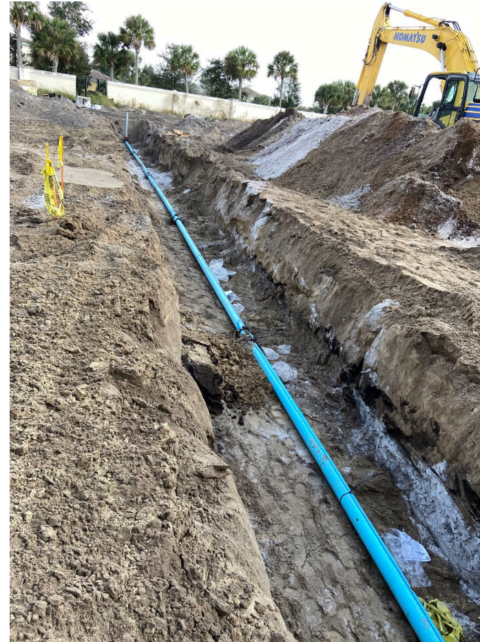
Installation of Main Water Line
