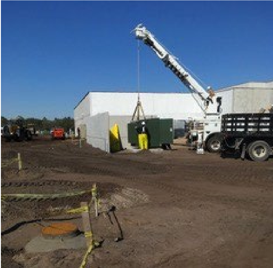
Transformer Placement
