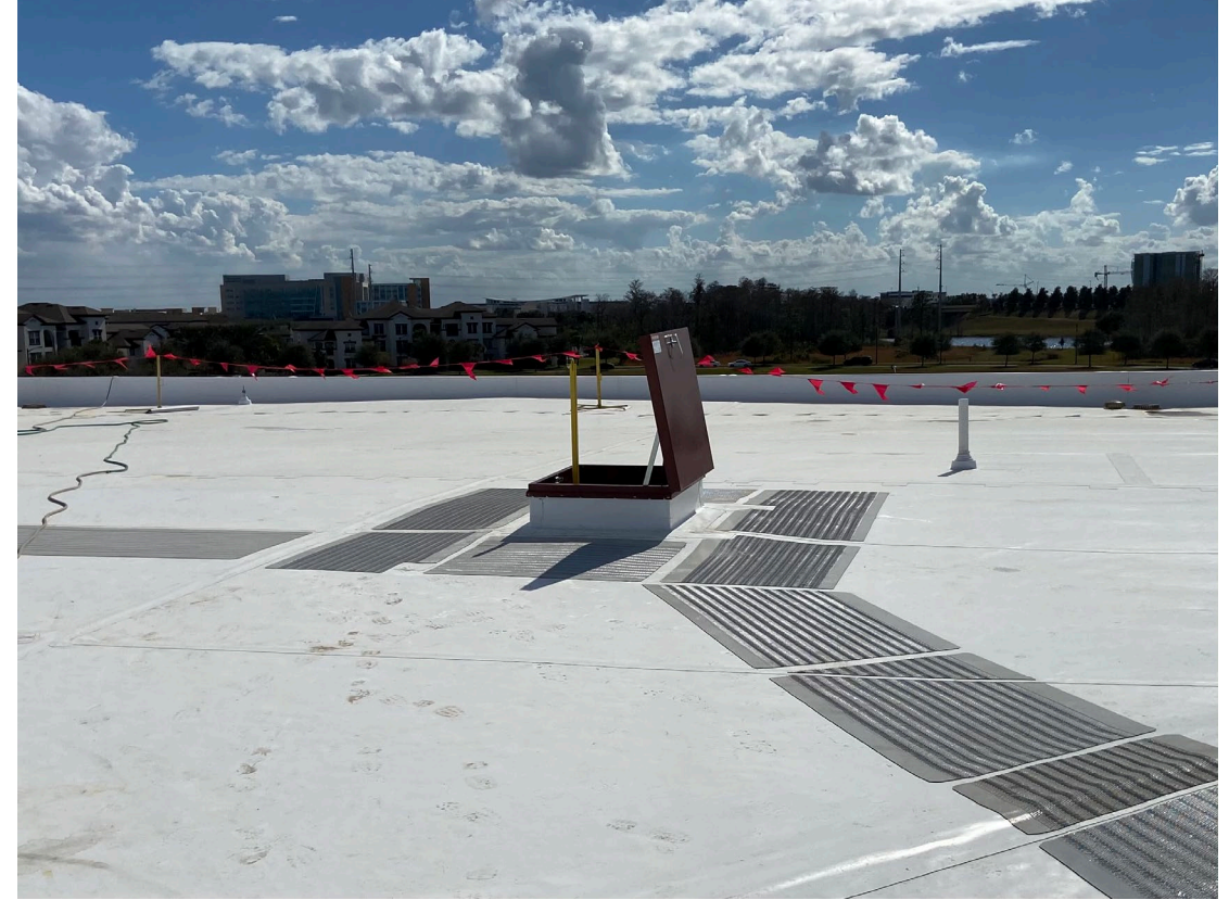
Roof Access Hatch
