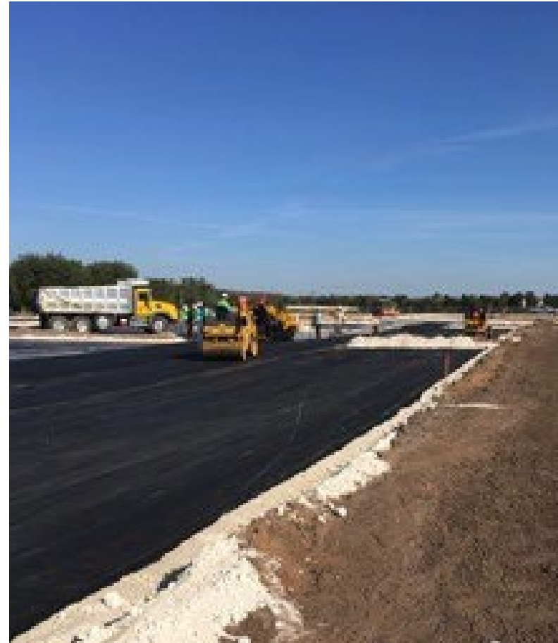
Asphalt paving for Parent Parking
