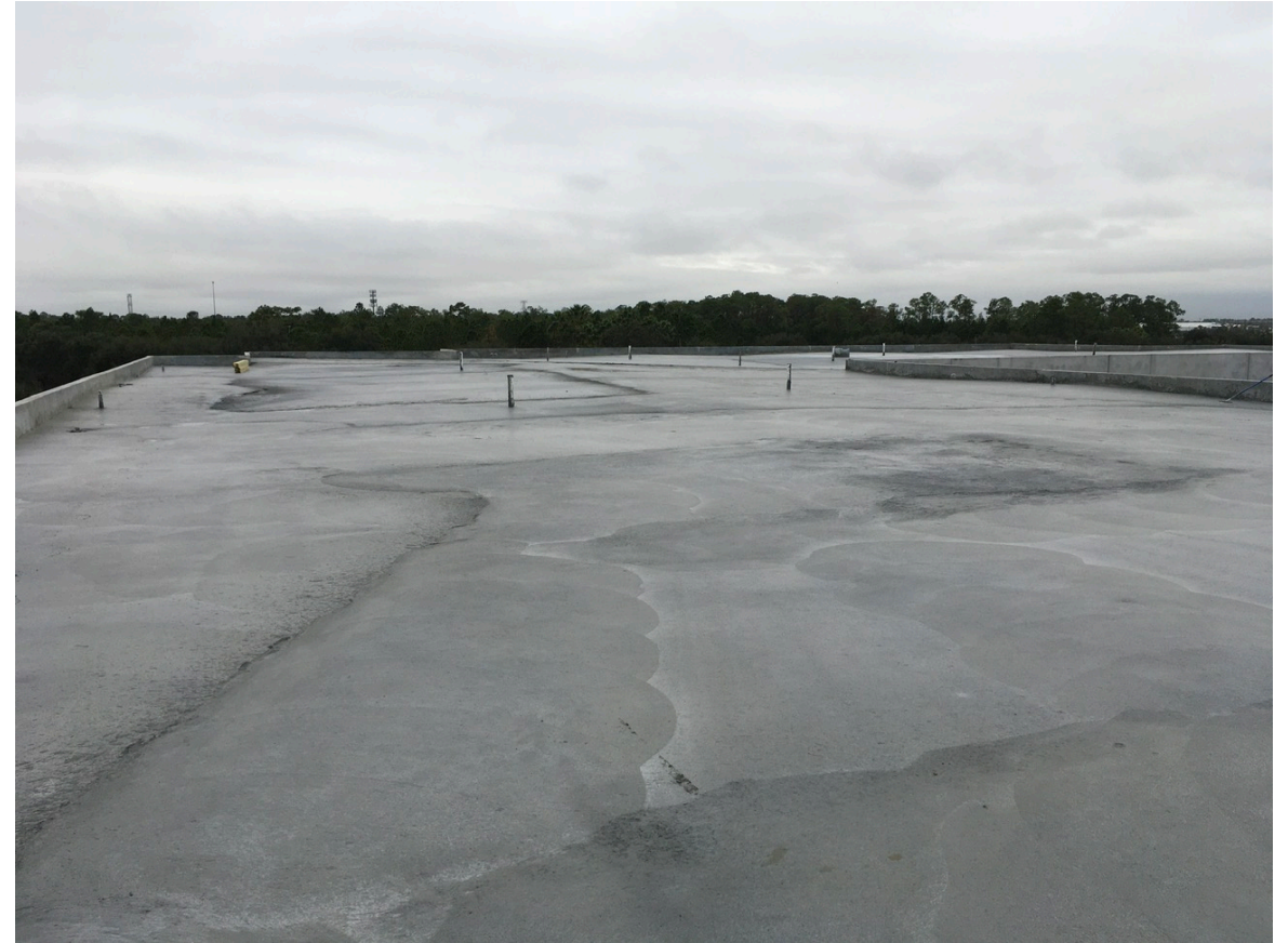
Lightweight Insulating Concrete
