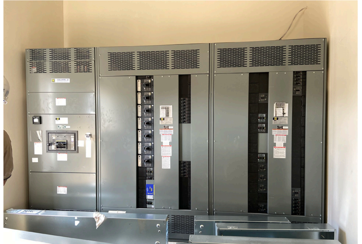
Building Main Electric Panel
