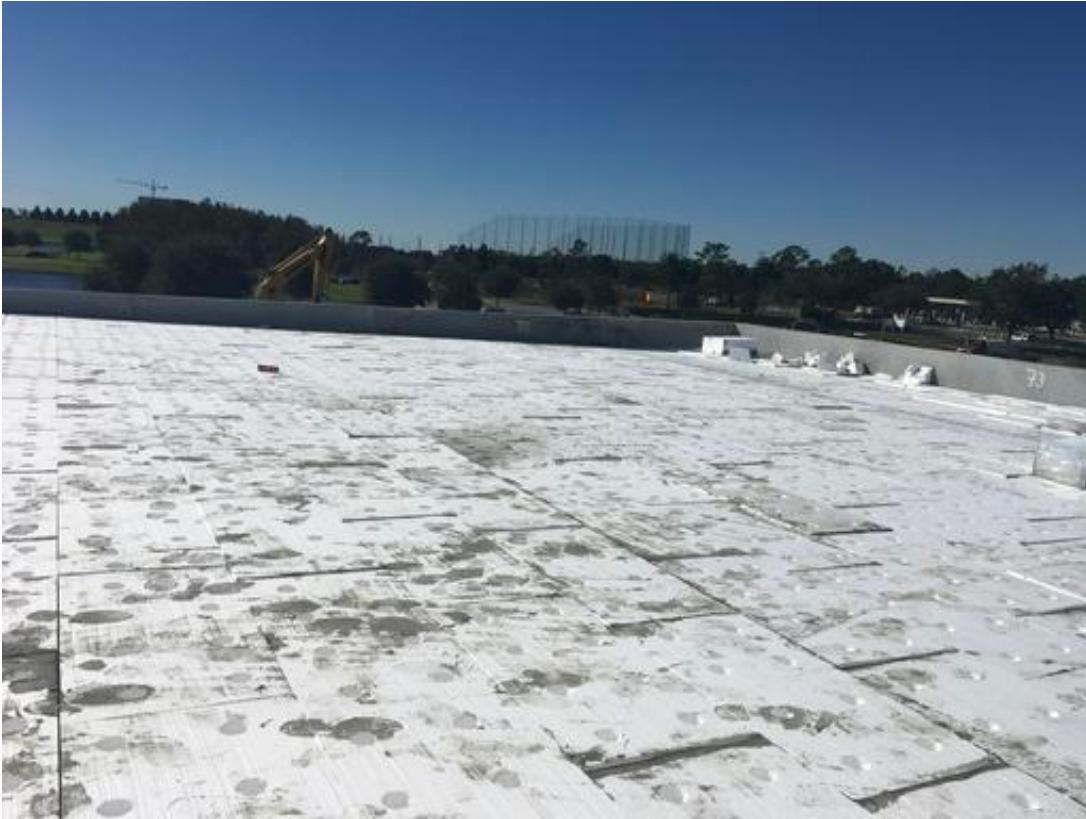
Foam Roof Insulation
