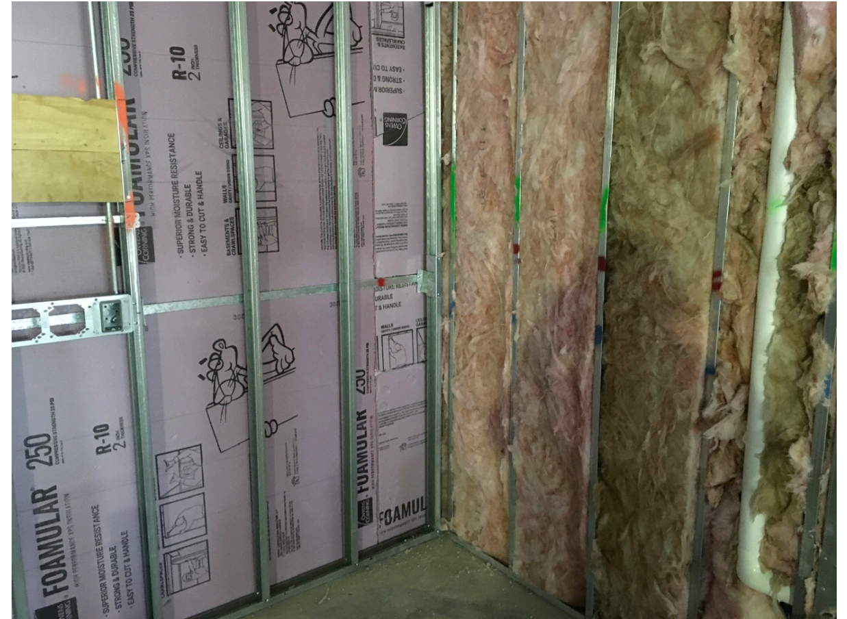
Interior Wall Insulation
