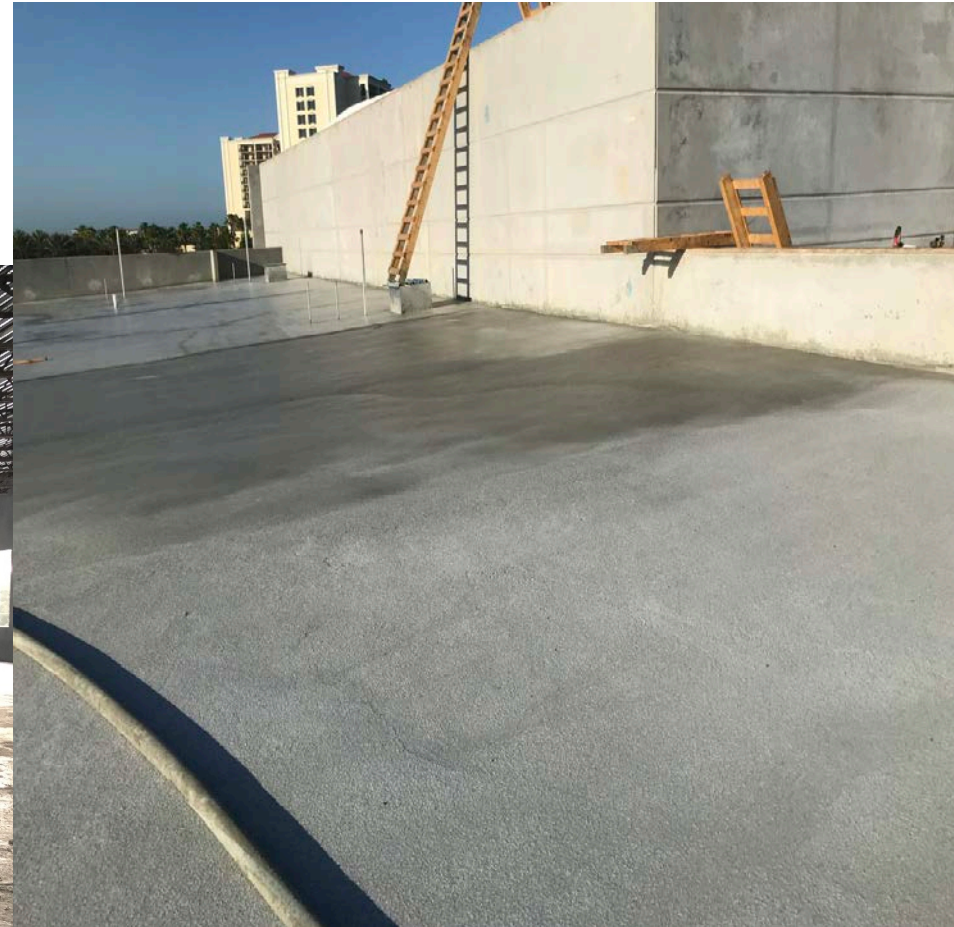
Installation of Roof Insulation and LWIC
