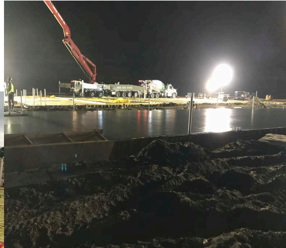
Pouring of Tilt Panels with a Boom Pump
